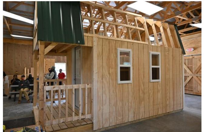
**Figure 4.** The nearly-completed cabin, constructed by students at Boys Home, is ready to be deconstructed, transported, and reconstructed on the chosen site on the mountain property behind the main campus. Mr. Sarratt and the students specifically designed the cabin in a modular design to enable initial construction inside the Trades Building.
